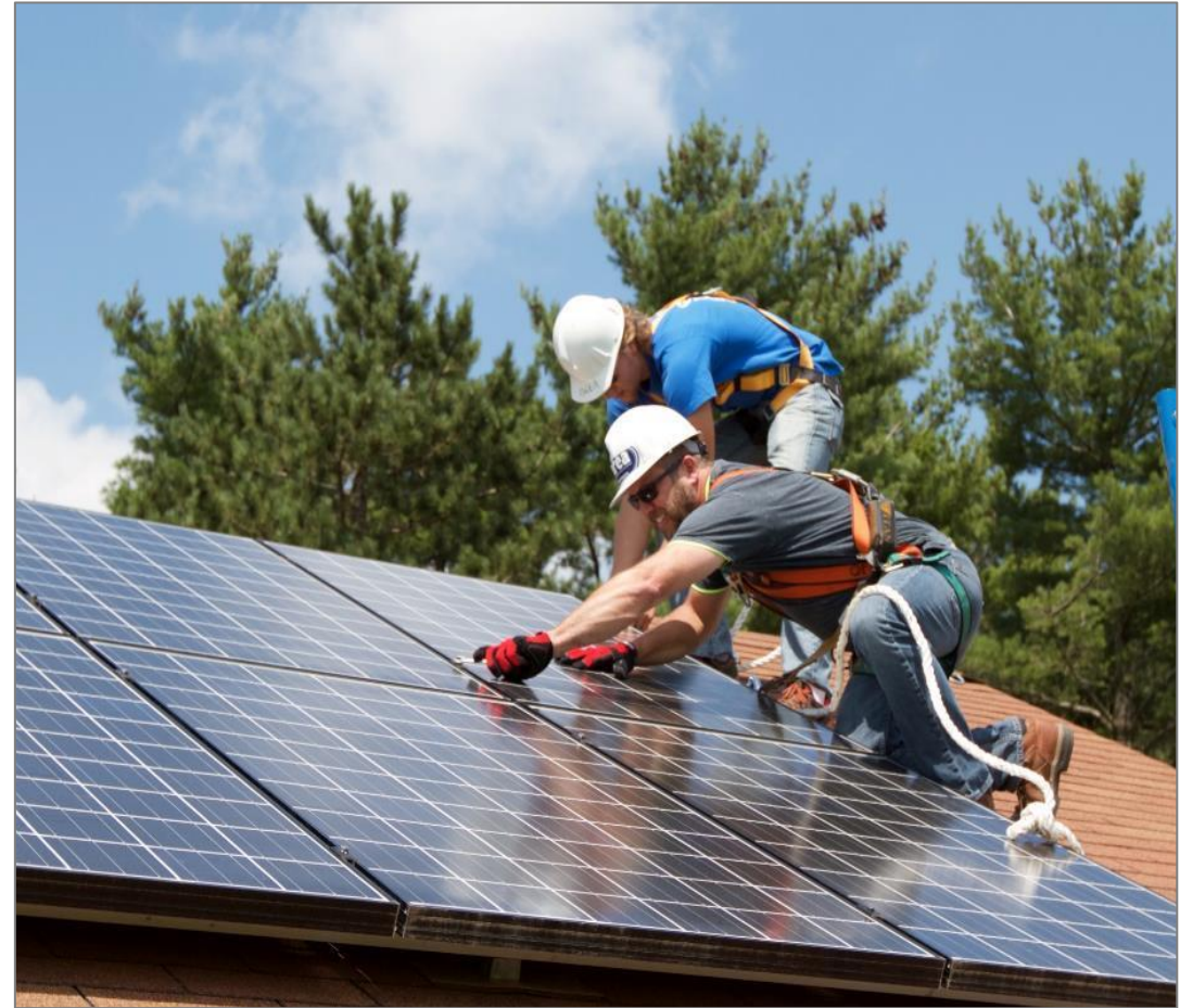
Installers configuring a roof-mounted system.
